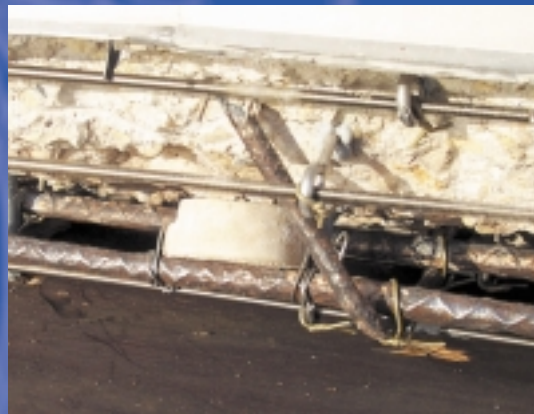
Galvanic Anode in a mortar shell is tied to the reinforcing bar before concrete patch is poured. The anode deteriorates in place of the embedded steel and thereby protects the concrete.
