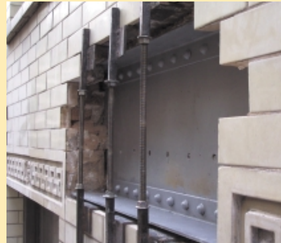
Above: Bracing support system at 28 East Jackson
