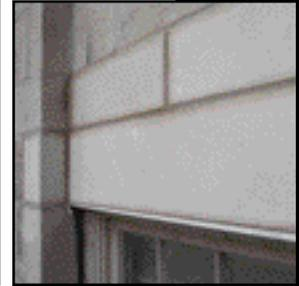
As discussed in earlier issues of this publication, corners are especially susceptible to deterioration. In the case of the Montgomery Ward Building, there are some small outcropped areas, irregularly shaped with numerous corners, requiring special attention. Corner replacements must be completed with care, as stability of the remaining pieces cannot be compromised.
