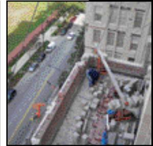
Even with numerous stones removed, the wall remains stable and weather tight. This can only be accomplished with proper planning and careful execution. Remaining stones are braced and openings are sealed against wind and rain.
