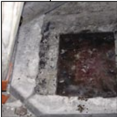
After the shoring was in place and the section of pier removed, the top of the beam was exposed. This beam runs under the sidewalk. Many areas of the city have roadways or work areas underground.
